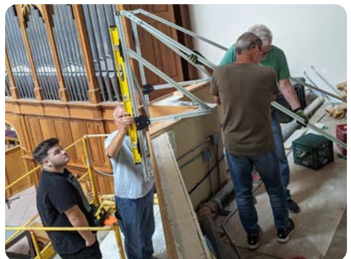
Dedicated Tech Team volunteers installing mounting brackets for new sanctuary screens.
