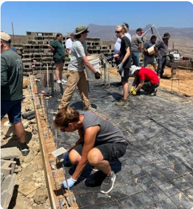
Hard at work preparing the foundation.
